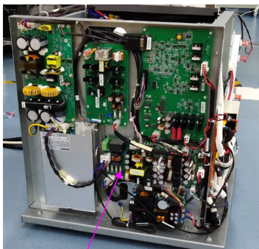
Auxiliary power board
